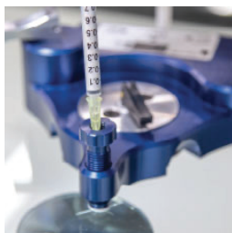
Step 2: Fill the chip with resin and then use the vacuum puller to add pressure to the repair area.
